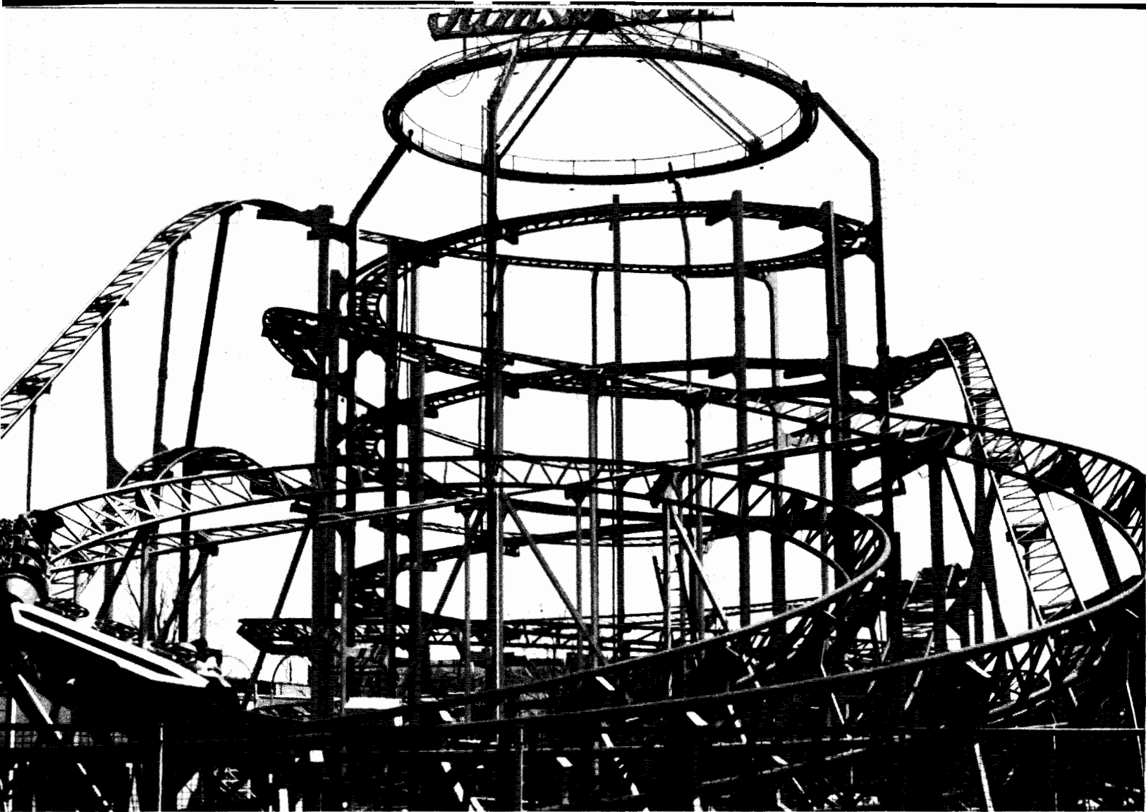
Figure 1. The Jumbo Jet at Coney Island, New York. An example of a horizontal loop.
